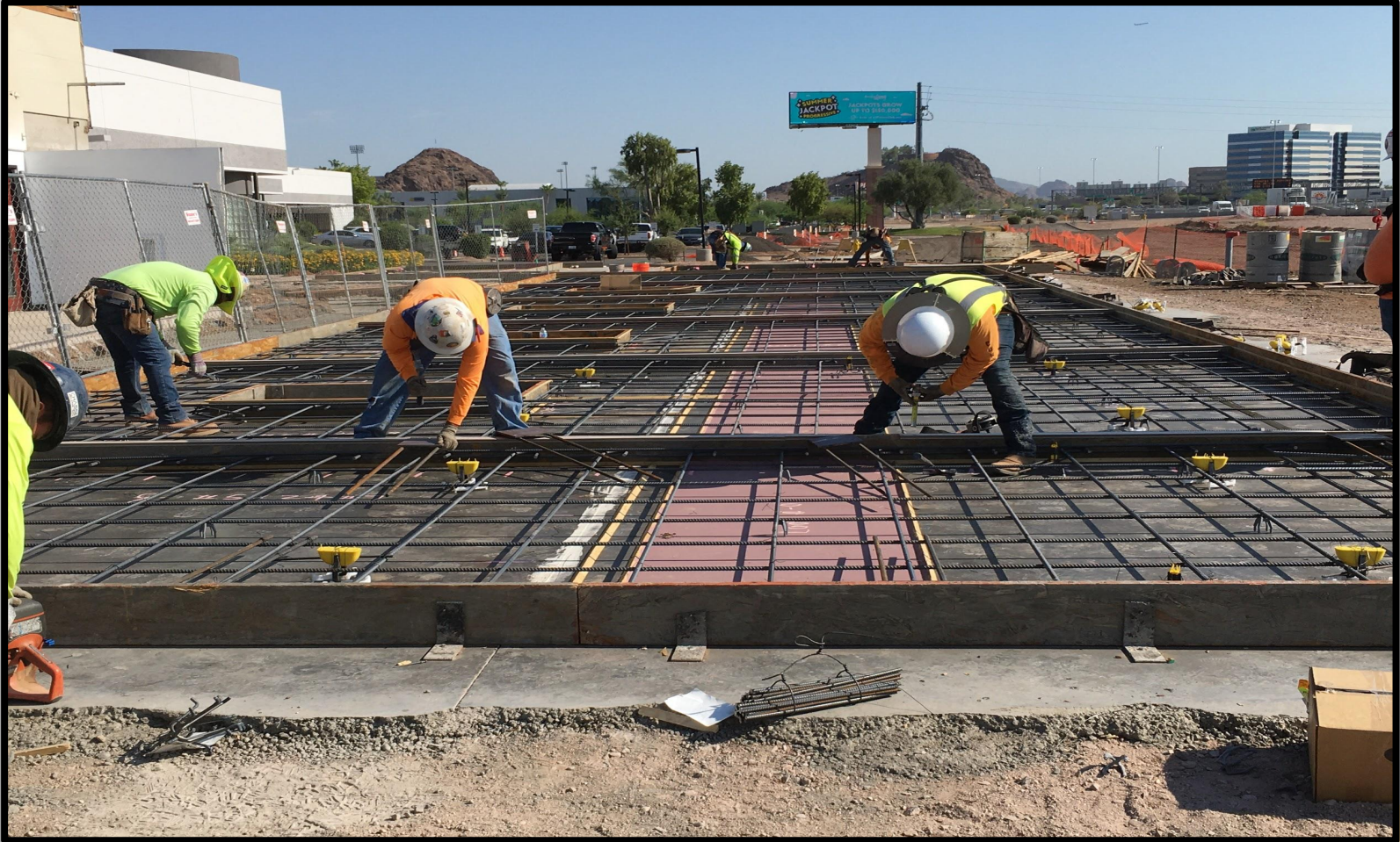
Rebar for tilt ups.
